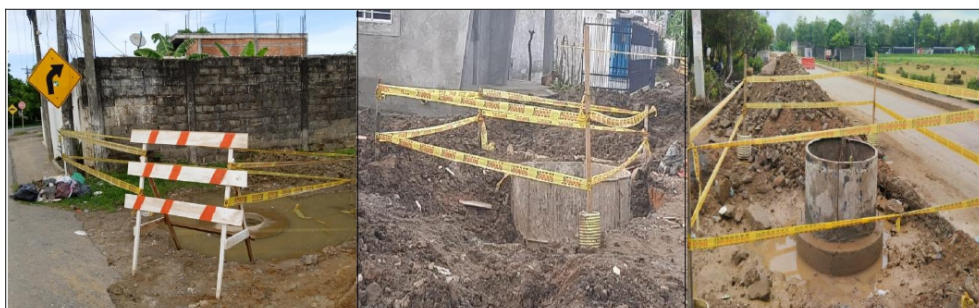
CERRAMIENTO A MANJOLES
