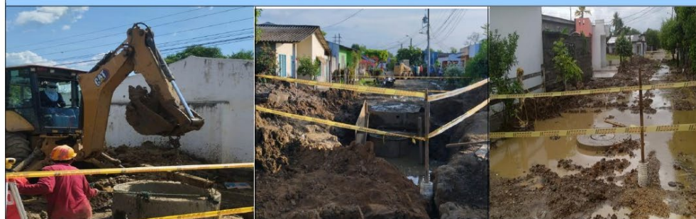
CERRAMIENTO A MANJOLES
