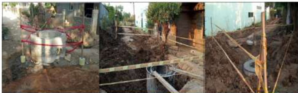
CERRAMIENTO A MANJOLES
